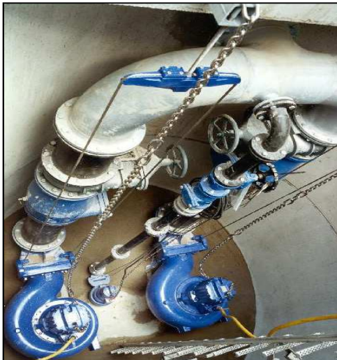
Pump chains (e.g. lifting or lowering pumps in fluid media for maintenance purposes) of nearly any dimension
